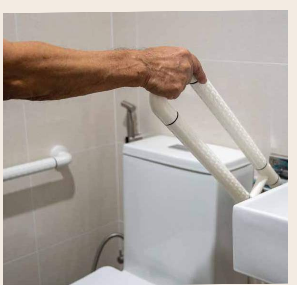
EASE Improvements: New grab bars to enhance the safety and comfort of seniors
